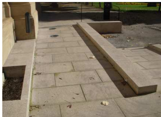
Access ramp to the Museum of Fine Arts.
