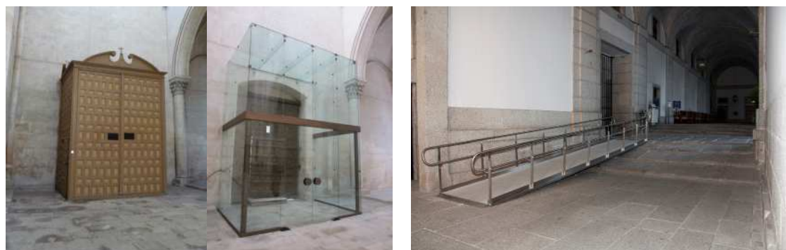
Before and after replacing the wooden porch with a glass windbreak at Las Huelgas Monastery.
