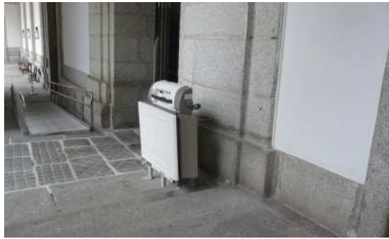
Platform lift in Patio del Abrevadero.
